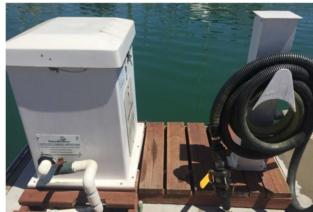
Motorized dump station requiring the manual opening of its ball valve for drainage
