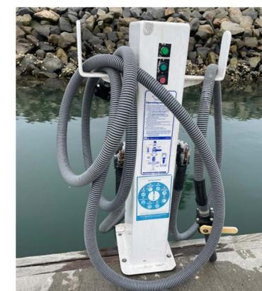
Pumpout unit retrofitted with a port-a-potty wand attachment
