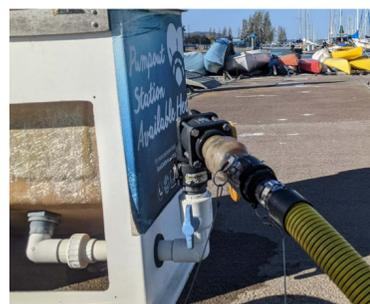
A gravity-drained dump station manually connected to a pumpout unit’s infrastructure by attaching the pumpout unit’s hose to the dump station waste fitting
